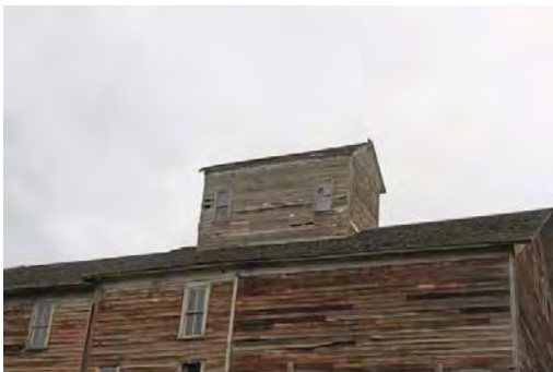
Head House Located Atop the Elevator Addition Looking North.jpg
