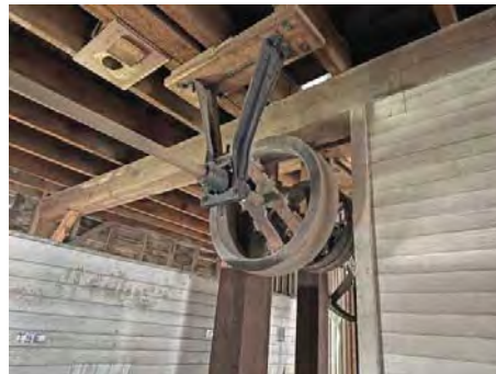
2nd Floor Main Mill Belt Wheel Assembly Looking NW.jpg
