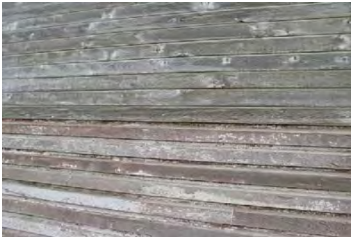
Mixed Siding of Ship Lap/Dutch Lap on Warehouse Structure.jpg
