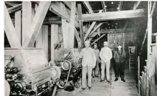
Interior Of Flour Mill ca 1910.jpg
