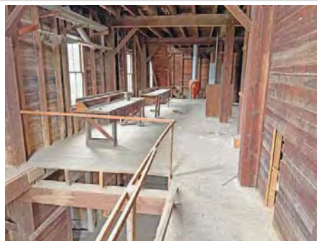
2nd Floor of Main Mill Workshop Area Looking East.jpg
