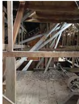
Distribution Chutes from Head House to Storage Bins Looking East.jpg
