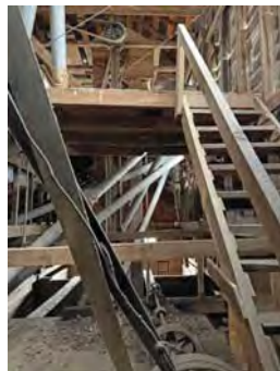
3rd Floor Stairway To Head House Showing Metal Distribution Piping Looking East.jpg
