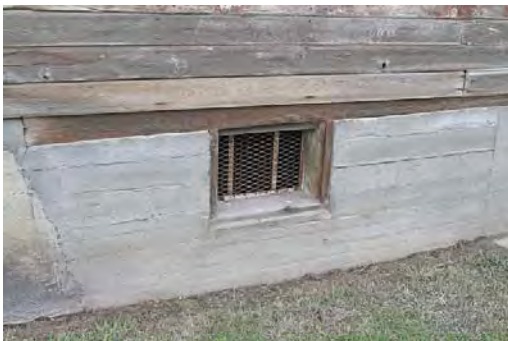
Window at Basement Level of Elevator Structure NE Elevation.jpg
