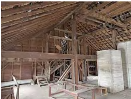
3rd Floor of Main Mill Looking Towards Stairway to Head House Looking East.jpg
