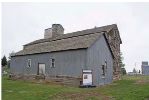
Grain Warehouse Structure Looking SE.jpg
