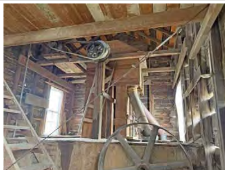
Head House Atop Elevator Addition Looking East.jpg
