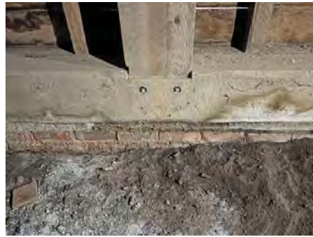
Brick Foundation Main Mill with Timber Bottom Sill Looking South.jpg
