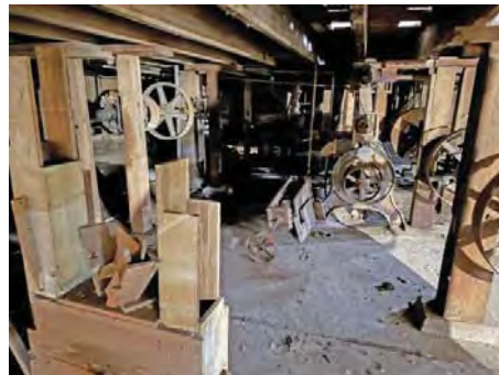
Basement Level Belt: Flywheels Looking East.jpg
