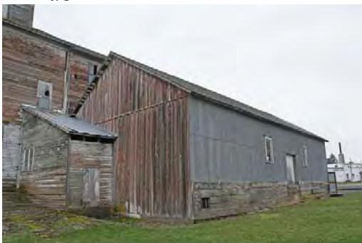
NW and NE Elevation of Warehouse and Smaller Dust House Looking SE.jpg
