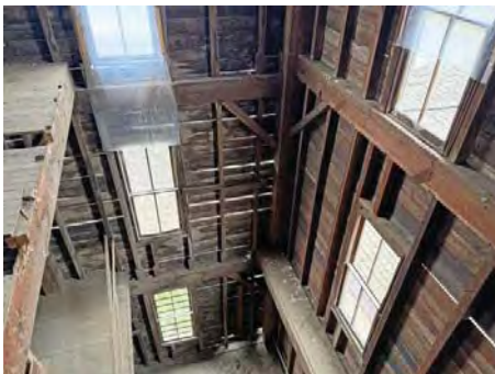
NW Corner of Main Mill Looking Down to 1st Floor NW Corner.jpg
