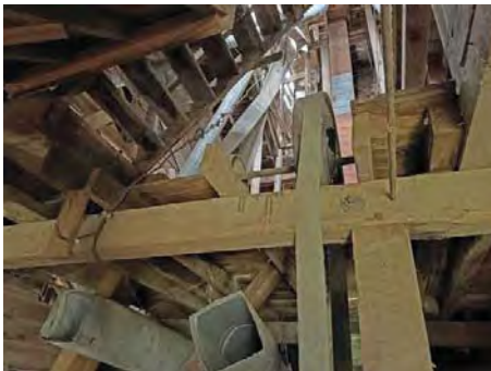
Belt Assembly and Stairway Looking Towards Head House.jpg
