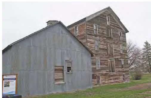
Northwest Elevation of Mill Proper and Warehouse Structure.jpg
