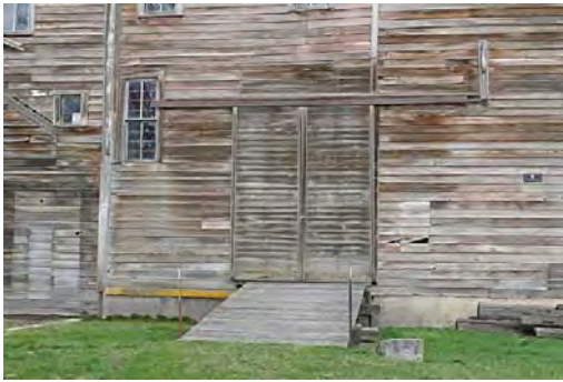
Exit/Entry with Ramp Leading Into Elevator Structure Looking North.jpg
