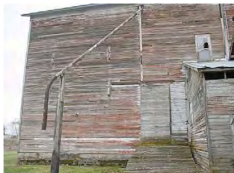
Grain Discharge Chute Looking South.jpg
