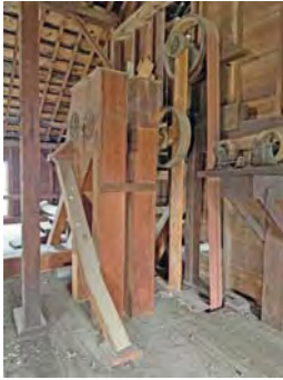
3rd Floor Level Grain Collector Housing Elevator Section Looking North.jpg
