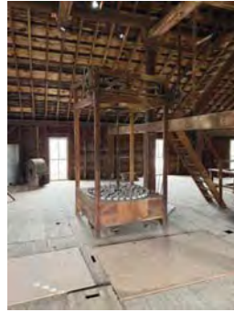
3rd Floor Disassembled Dust Collector Main Mill Looking South.jpg
