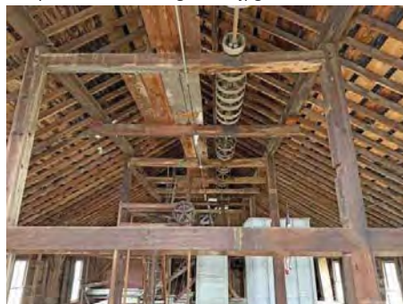
3rd Floor Level Wheel House with Heavy Timber Bracing Main Mill Looking East.jpg
