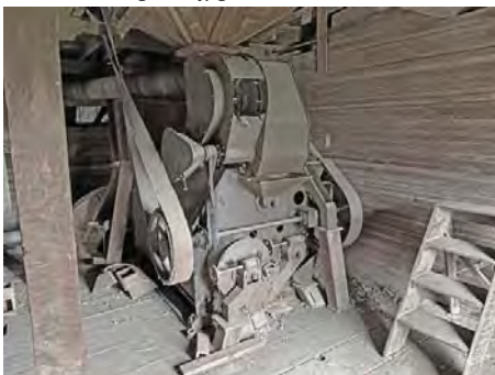
3rd Floor Main Motor and Hopper Top of Elevator Looking North.jpg
