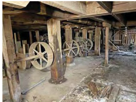
Basement Level of Main Mill Showing Post and Beam Construction and Basement Wheel House.jpg
