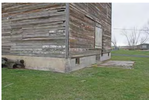
Foundation Detail at Elevator Structure Looking North.jpg
