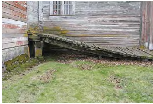
Exit/Entry Ramp at NW Elevation.jpg
