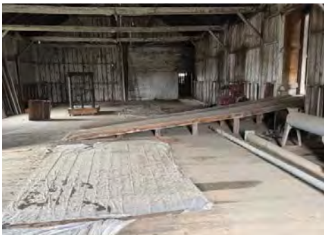
Warehouse Structure Looking East.jpg
