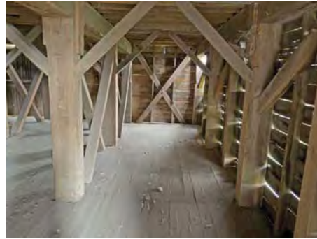
Interior SE Corner Main Floor of Elevator Structure.jpg
