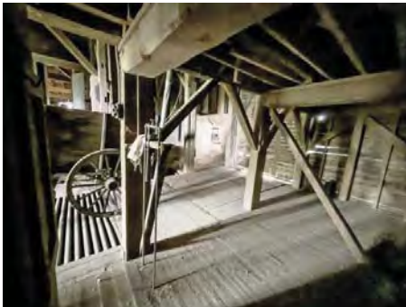
Elevator Lower Level Showing Pit Looking West Toward Main Mill copy.jpg
