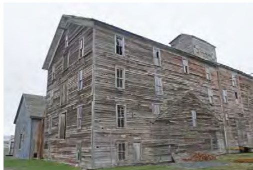
NW and SW Elevations Looking NE.jpg
