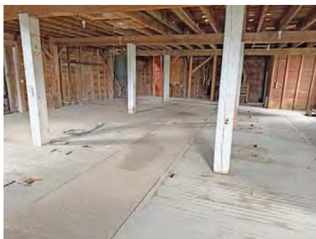
1st Floor of Original Mill Looking East.jpg
