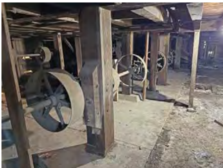
Basement Level Belt Wheels Looking NE.jpg
