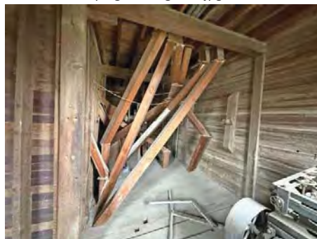
3rd Floor Multiple Wood Clad Metal Disbursement Chutes Atop Elevator Looking North.jpg
