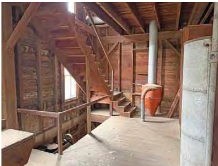
2nd Floor Stair Case Leading to 3rd Floor Level of Main Mill Showing Water Tank and Dust Collector at Foot of Staircase Looking NE.jpg
