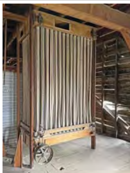
2nd Floor Dust Collector in Main Mill Looking SE.jpg
