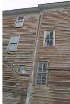
Elevator to Mill Proper Addition Junction Looking North.jpg
