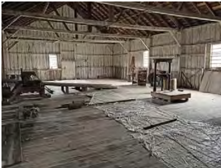
Interior of Warehouse Structure Looking West.jpg
