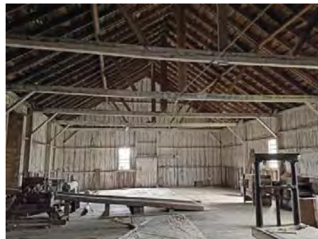
Warehouse Structure Showing a Scale and Two Fanning Mills at the Far Right Looking West.jpg
