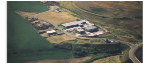
The Pullman Industrial Park in its early stages, 1980s
