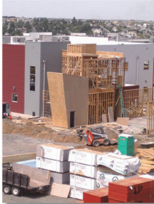
Construction at PIP, 2000s
