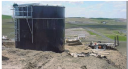
Water tank construction at Colfax Industrial Park, 1993
