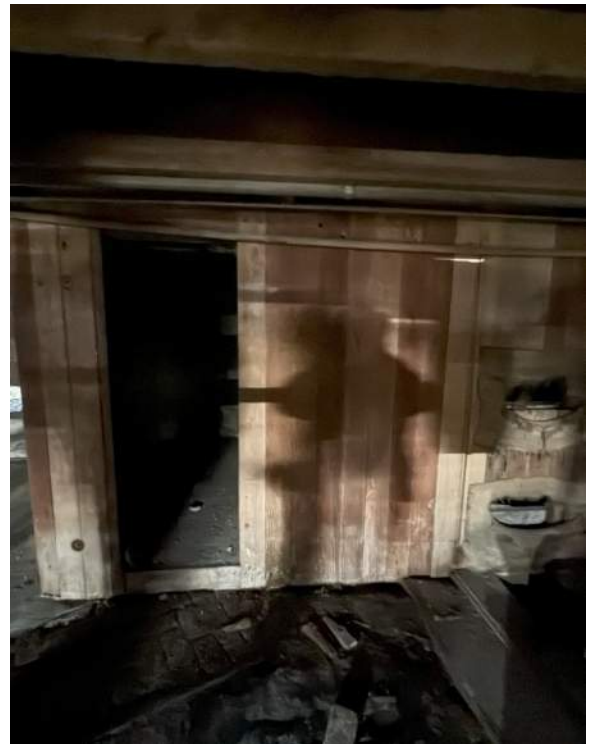
Motor Room looking north.
