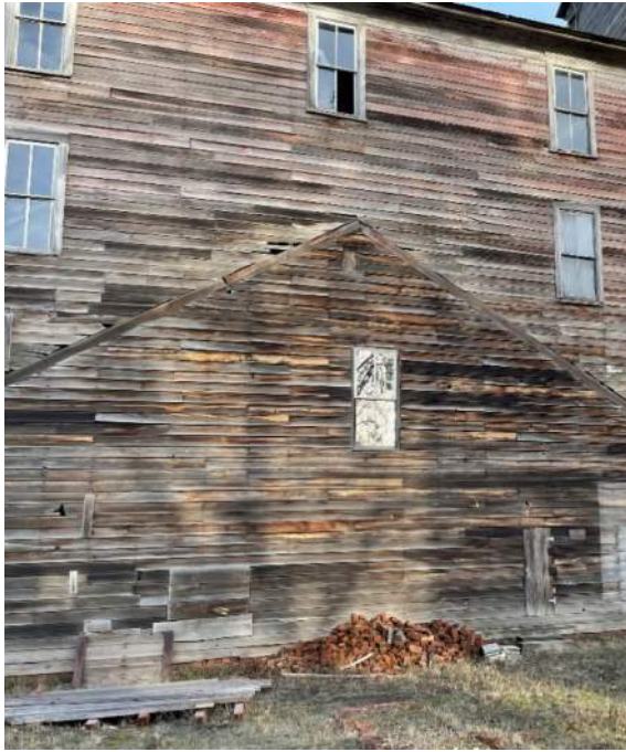
Former building addition location looking north.
