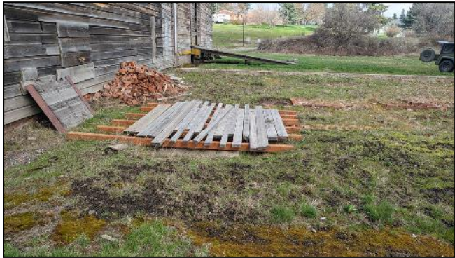
Photograph 3: View of the scale and loading door on the east side of the mill, looking west.
