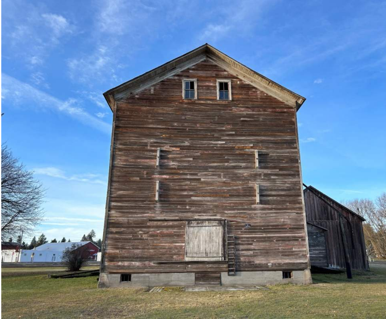
East side of existing J.C Barron Mill.
