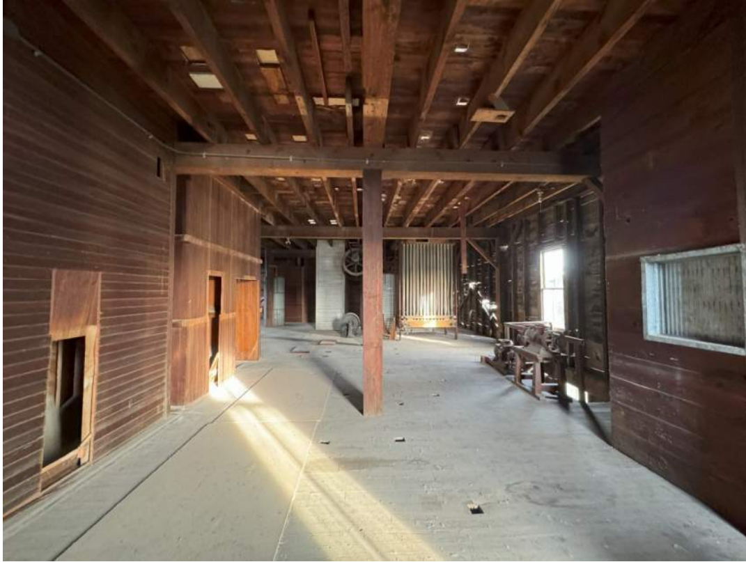
Second Floor Main Room facing east.
