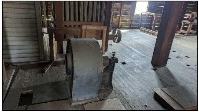
Photograph 8: Remnant infrastructure in the mill on the 2 nd floor.
