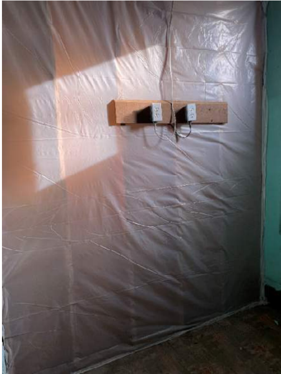
Safe Room new wall looking east.
