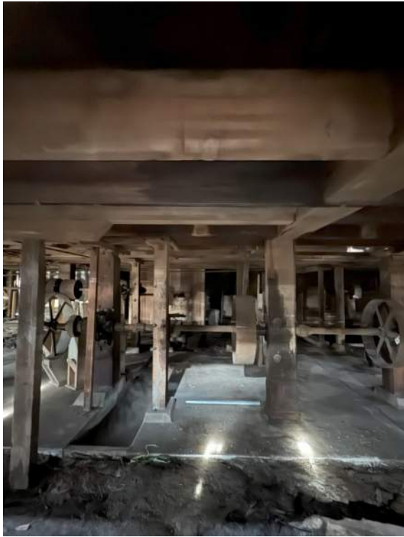
Basement looking north.
