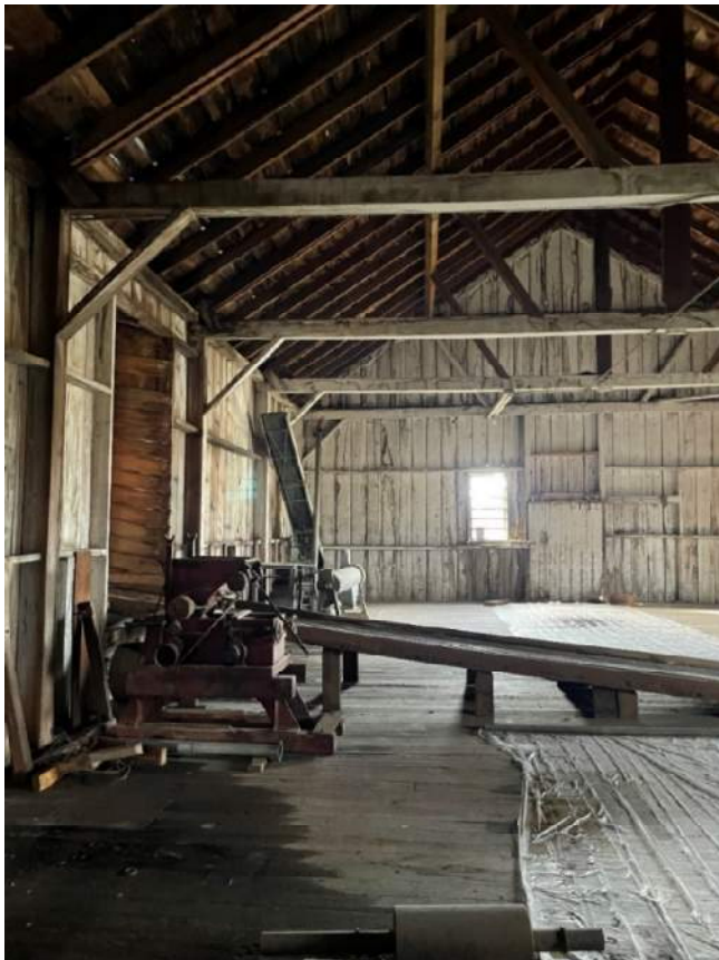
Flat house Image looking west.
