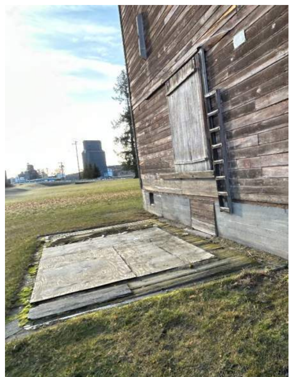
Plywood Covered Opening looking south.
