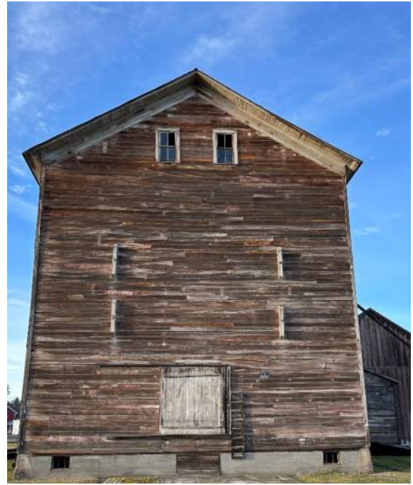
Façade looking west.
