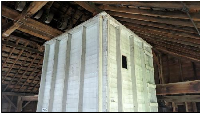
Photograph 9: View of a grain storage bin on the top floor of the mill.
