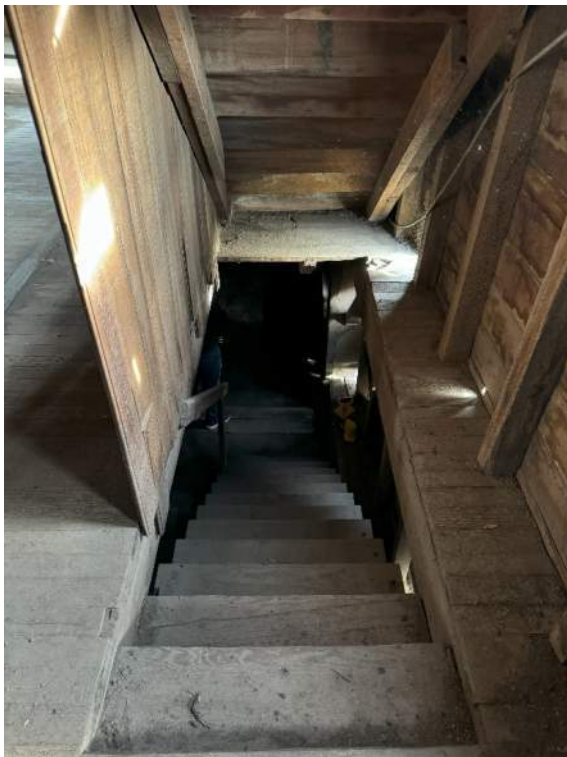
Basement Stairs looking east.
