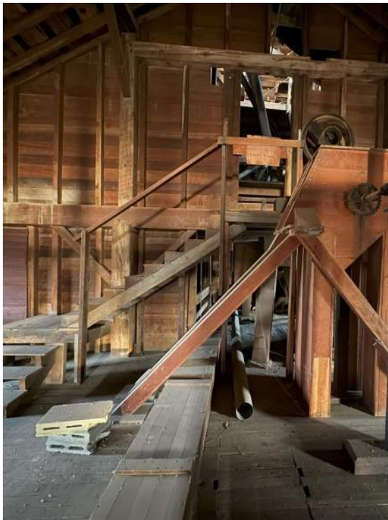
Stairs to Penthouse looking east.
