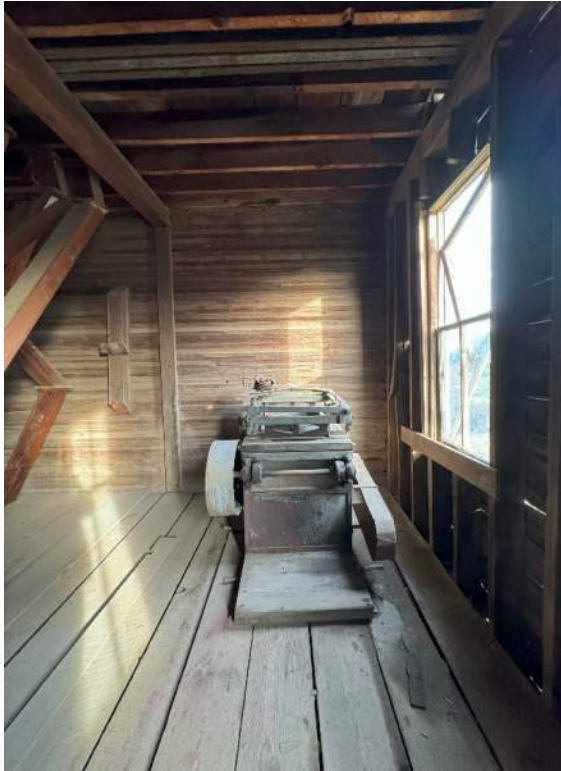
Equipment Room looking east.
