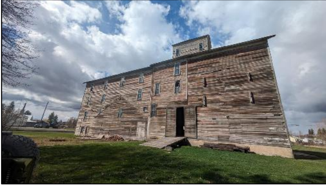
Photograph 1: View of the site's building from the south, looking north.
