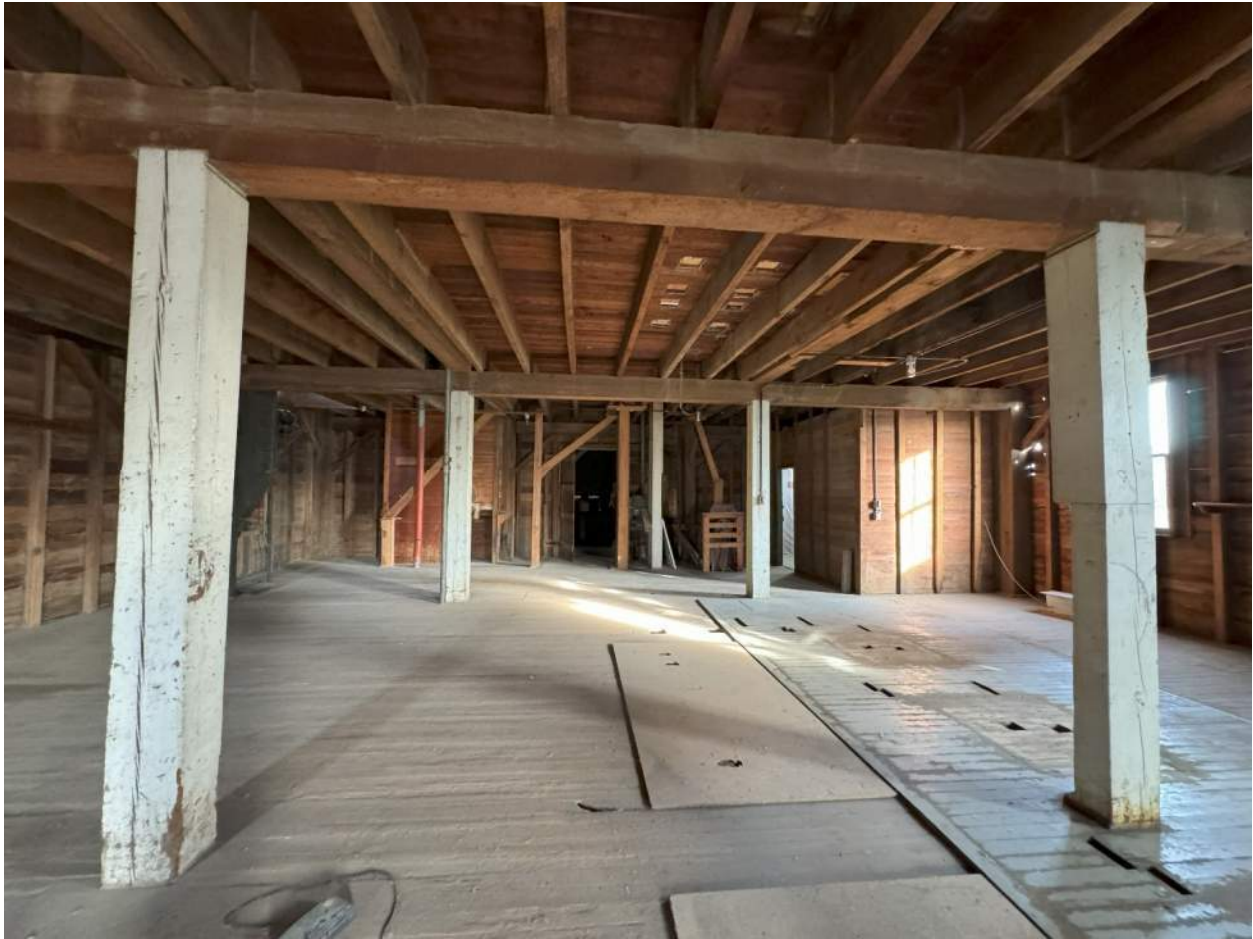
Interior Mill Image looking east.
