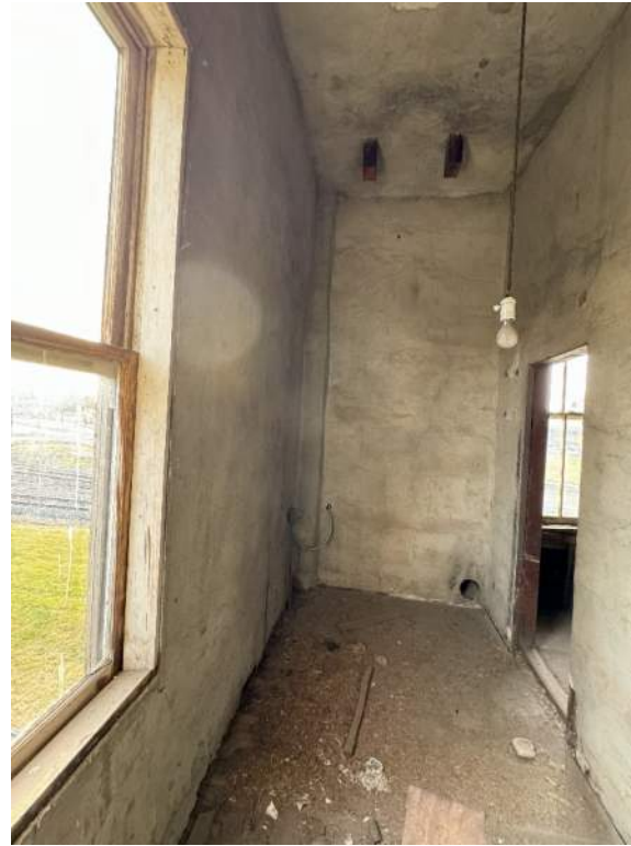
Plaster Room looking west.
