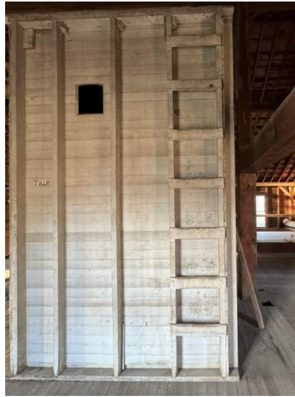
Framed Structure looking north.
