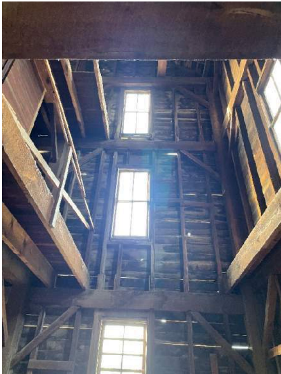
Three story opening from first floor looking west.
