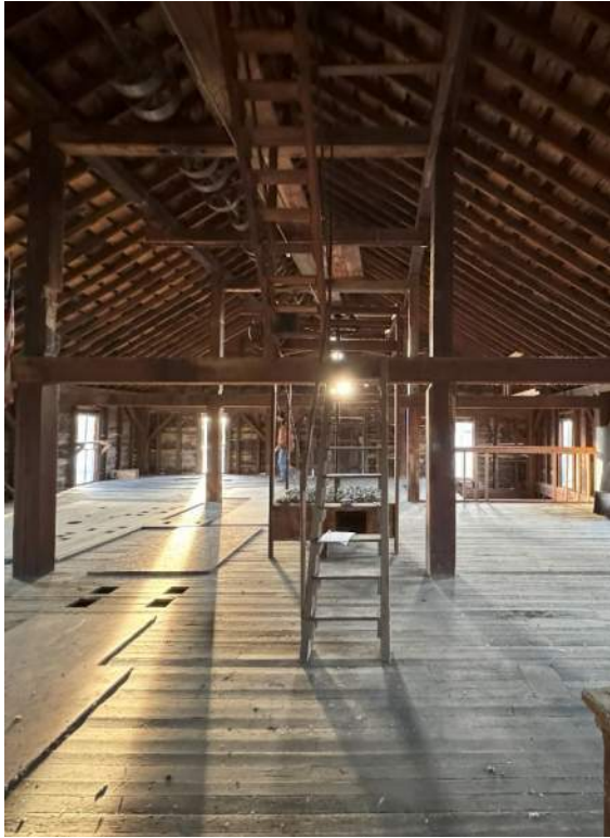
Main Room looking west.
